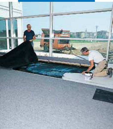
Installing industrial flooring in an electronics company
