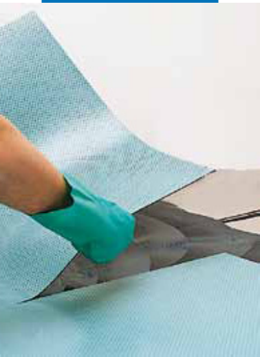
Laying conductive PVC tiles
