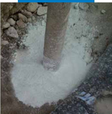
Application of Mapeproof Seal around through piping
