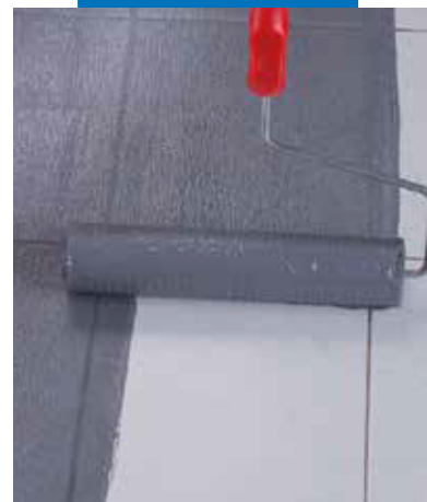
Application of Eco Prim Grip Plus by roller on existing porcelain tiles
