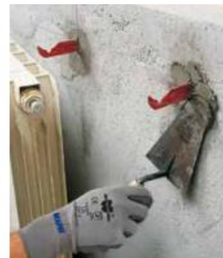
Fixing anchor bolts for radiators using Lamprocem
